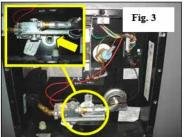
Water heater drain plug location
