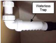
the internal seal that may potentially allow sewer gases to escape into the RV interior. The waterless trap can be unscrewed from the water lines. A label has been placed near the location of the waste valve that reads as follows:
