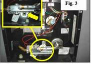
Water heater drain plug location
