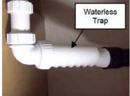
piping to open the drain. Passing a cleanout tool through the waterless valve may cause damage to the internal seal that may potentially allow sewer gases to escape into the RV interior. The waterless trap can be unscrewed from the water lines. A label has been placed near the location of the waste valve that reads as follows:
