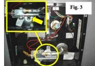
Water heater drain plug location
