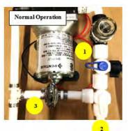
*Sanitize/Fill Tank*: Water from CITY connection or from SIPHON HOSE using the pump.
