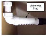
gases to escape into the RV interior. The waterless trap can be unscrewed from the water lines. A label has been placed near the location of the waste valve that reads as follows:
