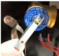
T&P Relief Valve Example
