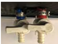
Low Point Drain Example
