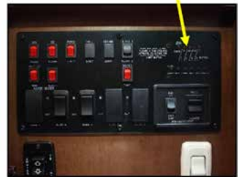
Monitor panel and command center panel
